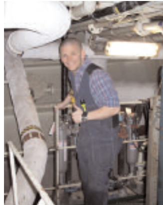
Electrical installation begins.
